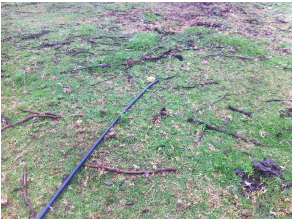
Photograph B16 Lawn sprinkler attached to effluent hose from septic tank.
